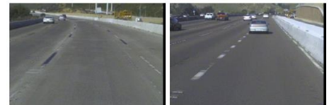
(c) Dark on light lane markings (d) A combination of segmented lines, circular reflectors, and physical barrier marking lane location
