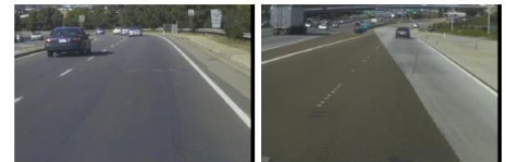
(a) A simple road with solid and segmented line lane markings (b) Circular reflectors and solid-line lane markings with non-uniform pavement texture
