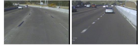
(c) Dark on light lane markings with circular reflectors (d) A combination of segmented lines, circular reflectors, and physical barrier marking lane location
