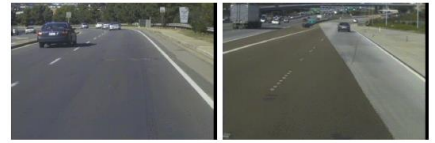
(a) A simple road with solid and segmented line lane markings (b) Circular reflectors and solid-line lane markings with non-uniform pavement texture
